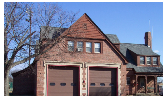
Pawtucket Fire Station 6, where the unconstitutional searches took place
